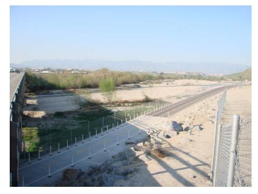
JBA performed a scour analysis and hydrology/hydraulics study for the Santa Ana River Channel at the Riverside bridge between the Ricks Facility and Riverside Avenue as part of the design of a cocomposting facility in Colton, CA. This stretch of the Santa Ana River channel has a calculated 100-year peak flow of 195,000 CFS and velocity of 27 FPS; it was therefore necessary to protect the channel
